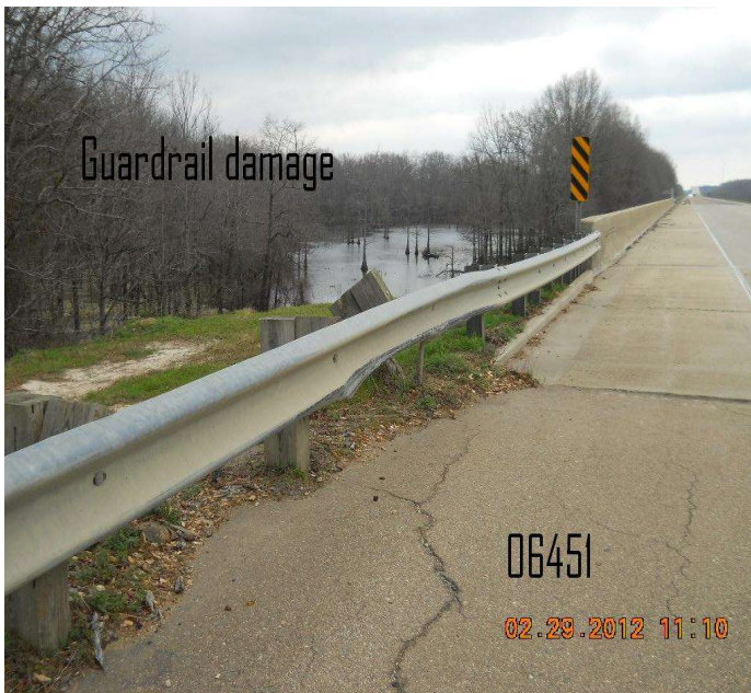
PHOTO 1 Description Abutment 1 Lt. Guardrail has old collision damage to the rail and post.
